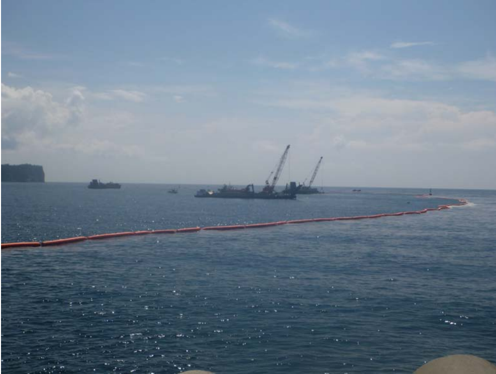
Figure 11. Barges placing fill or riprap on the sea floor at the construction site.
