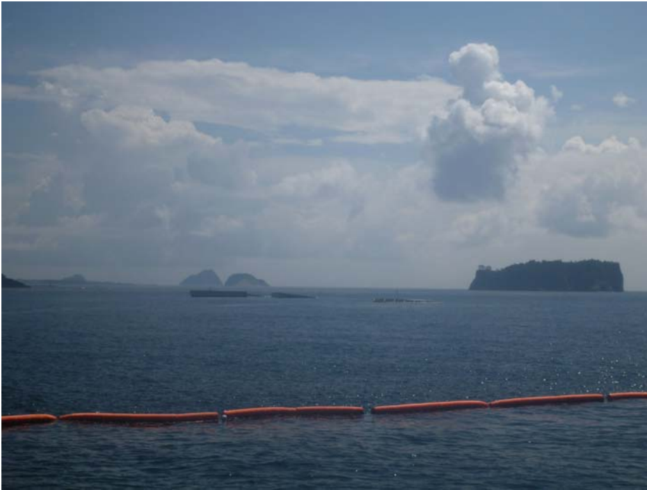
Figure 9. Silt screen around the base. Tiger Islet and floating caissons (since badly damaged by Typhoon Bolaven) can be seen in the background.
