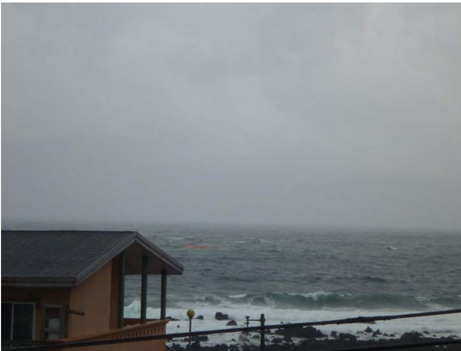
Figure 10. Silt screen torn loose from the construction site during moderately high seas on August 23 rd , 2012.
