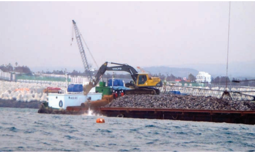
Image: Save Our Seas Construction workers dump unwashed rocks over the side of a barge, without a silt protector curtain or a fall pipe, completely ignoring environmental regulations, including their own mentioned in the Navy's EIA.
